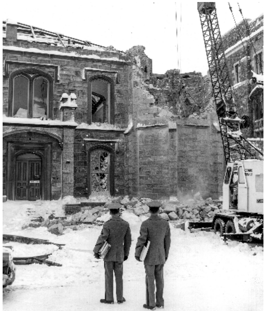
Bottom: Cadets watching the demolition of the Library in February 1962.
