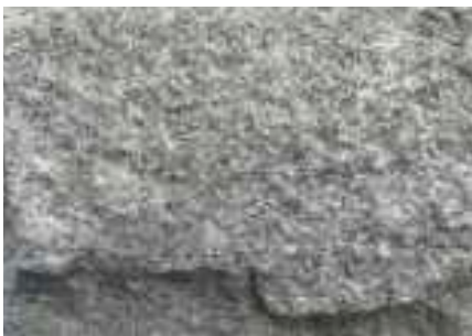
Top: Closeup of striated gneiss in the wall of the 1852 Central Barracks, now the Old 1st Division. PHOTO BY AUTHOR
