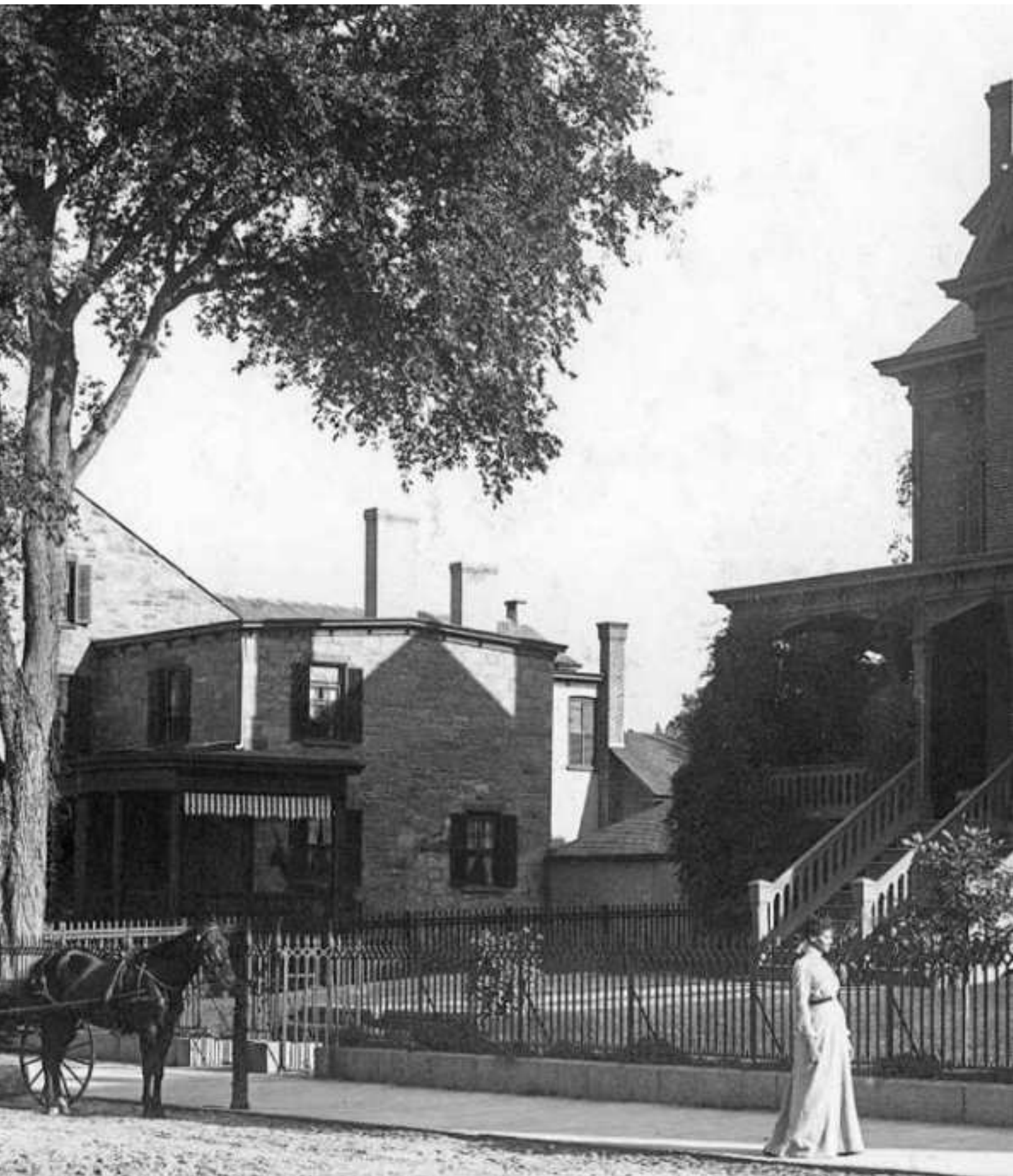
Quarters 39 & 41, dated to 1821, was the first of the stone duplexes to be finished. Today, they are Quarters 107a & 107b. This photo from 1902 shows a long iron fence that no longer exists. USMA LIBRARY ASC
