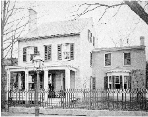
COMMANDANT'S QUARTERS, 1819. Some sources list this as completed in 1821, but building updates sent to the War Department in 1819 indicate it was completed that year just before winter set in. Thus, it is the oldest house at the Academy. Numerous modifications and additions have changed the original structure. This photo is from about 1870 and shows an added porch and addition on the right.
